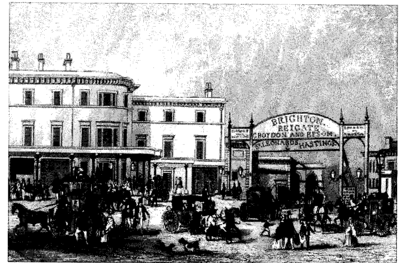
South Lasilrn Railway Station, London
