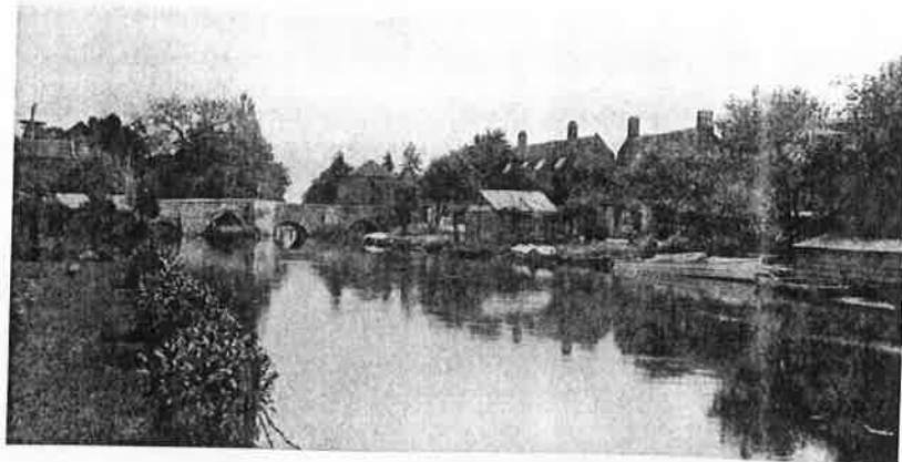
The River Ouse and Bridge in Brandon
